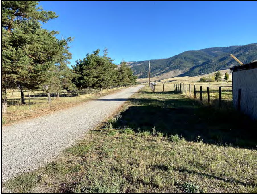
Photo 7: Representative view of a proposed pipeline route adjacent to a residential public roadway.
