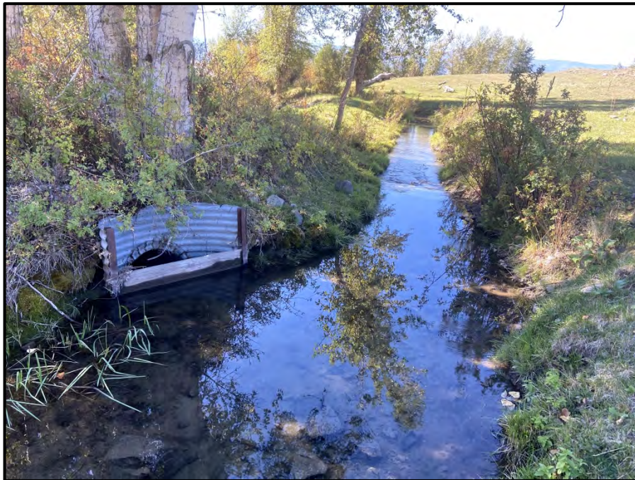
Photo 14: View of the inlet for supplying water to TRIB 2 directly from the K Canal.
