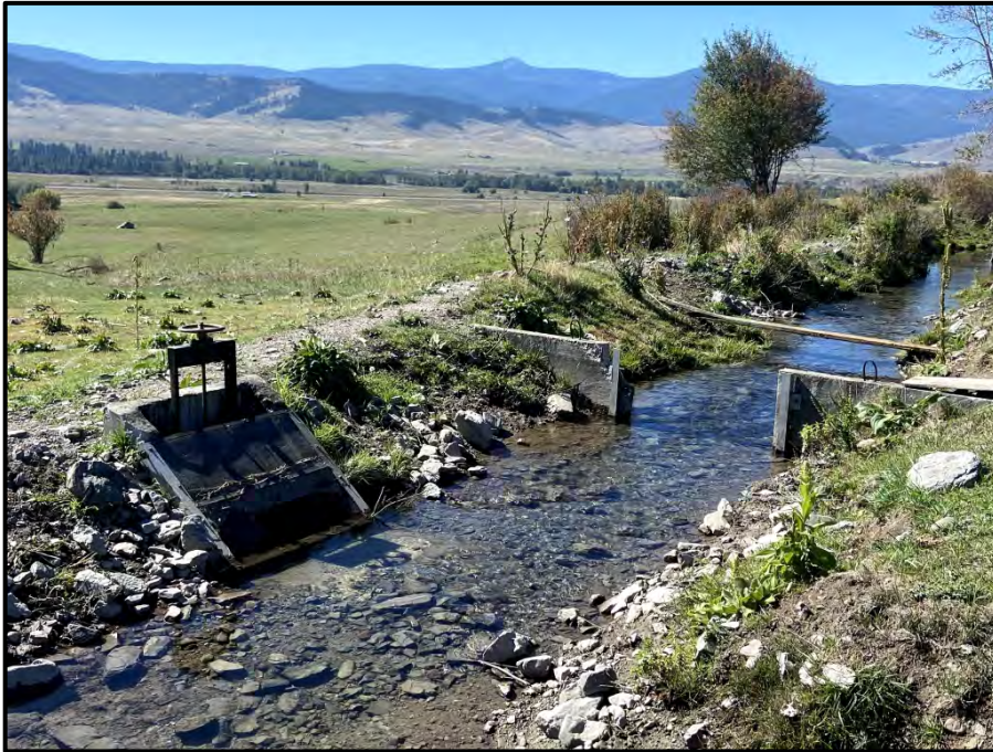
Photo 13: View of one of the many headgate structures on the K Canal.
