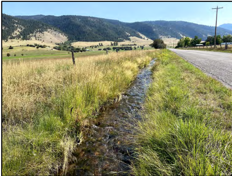
Photo 2: Representative view one of the existing irrigation ditches along the roadside that is proposed to be converted to pipeline.
